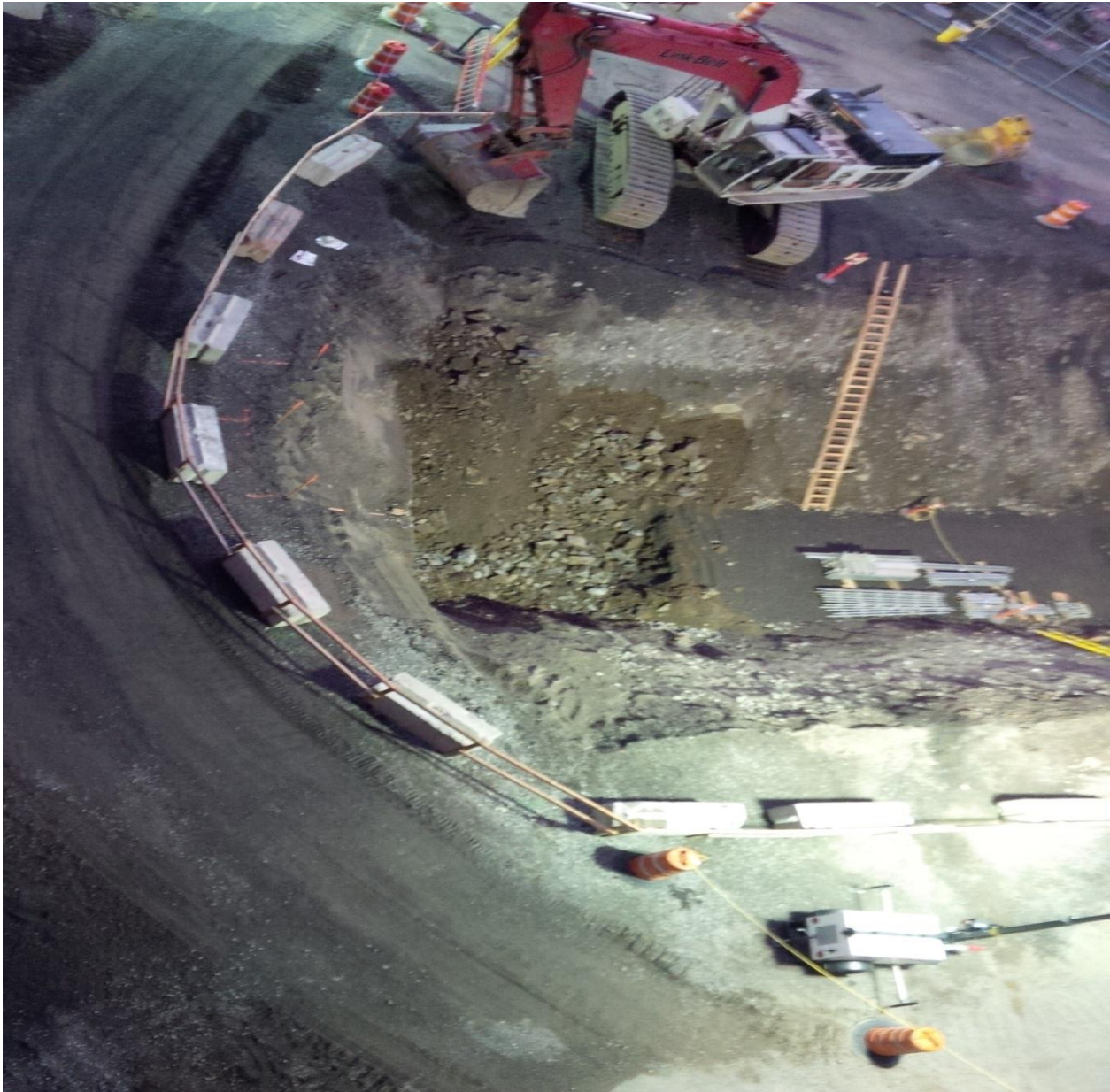
Small bedrock section that required rock hammer.
